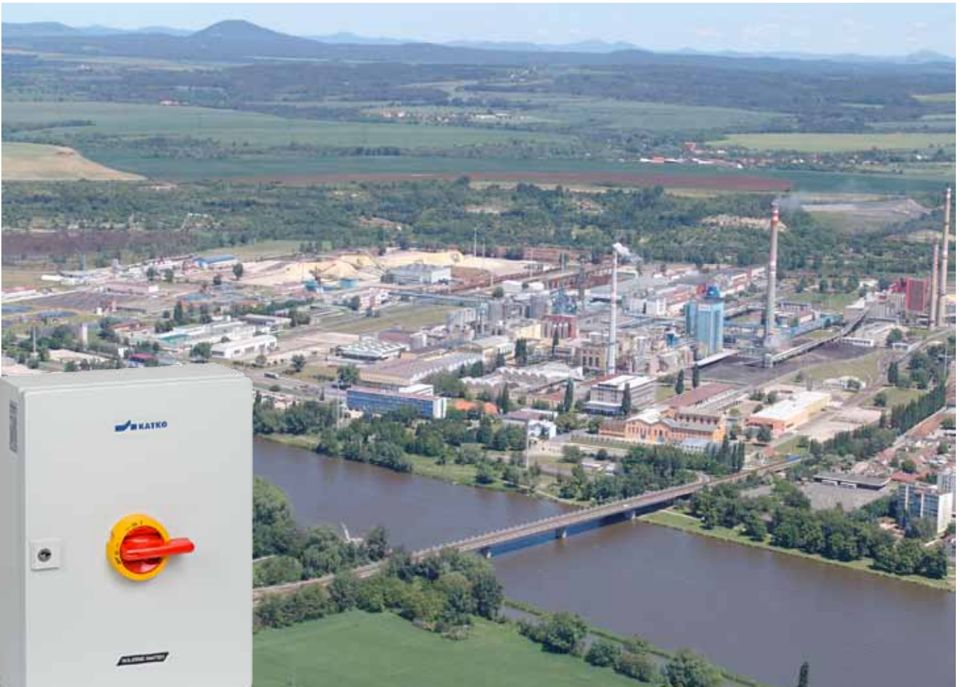
KATKO safety switches in Mondi Steti White Paper s.r.o., Czech Republic's largest Paper Mill, customer: Siemens Engineering Steti
